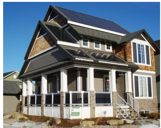
Figure : Building-Integrated Solar PV and Thermal
