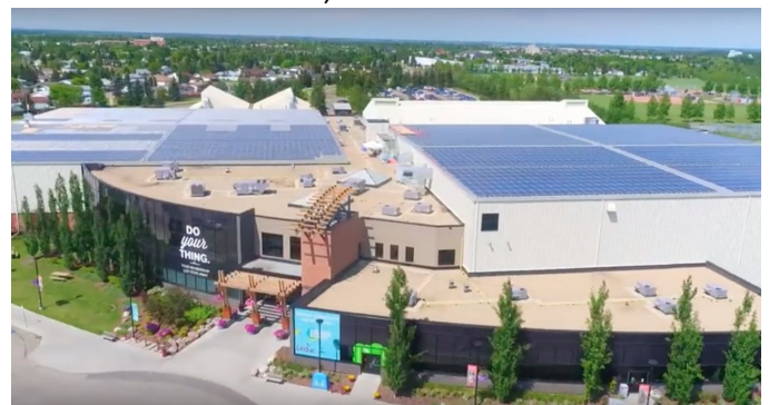
Figure 9: City of Leduc Recreation Centre
